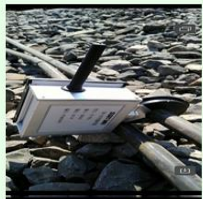
Lateral joint monitoring
